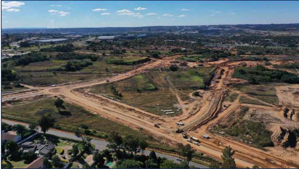
BDC- Installation of Bulk and Link - Roads
