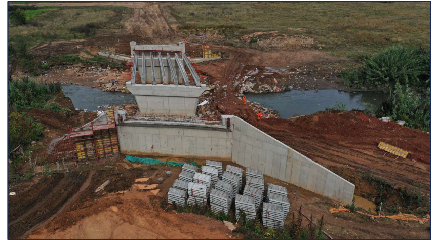
BDC- Installation of Bulk and Link – Bridge Construction
